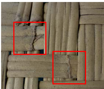
〈Fig. 27〉 Spliced Reed Joint in a Satgat (Photographed by Authors)
